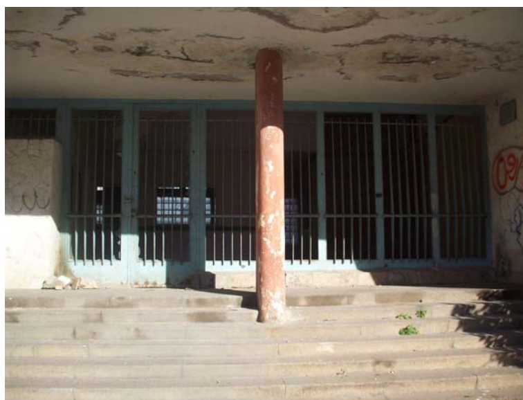
Exterior of Derb Moulay Cherif, former detention center in Casablanca.
